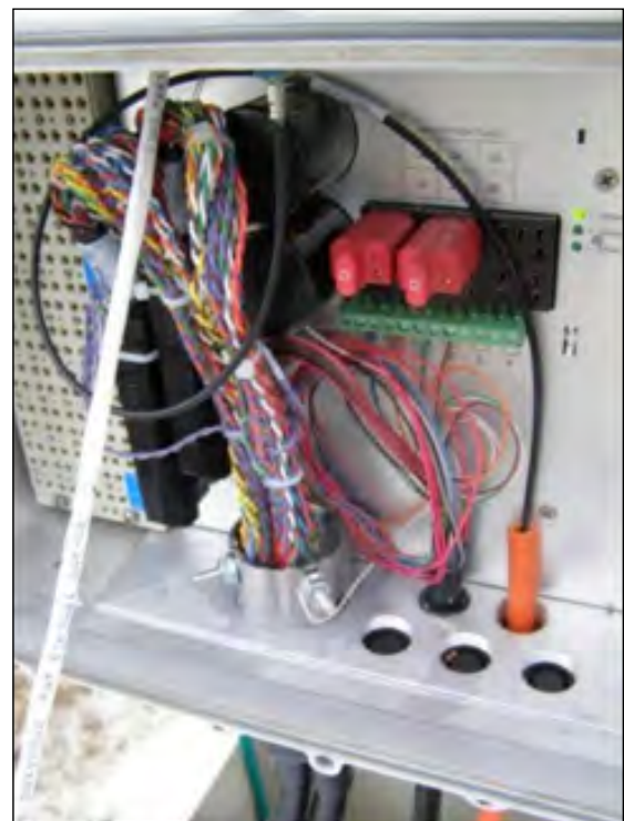
Figure 4 Typical DSLAM Terminal Strip
