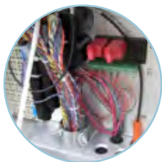
Figure 8: OSP Connections at the DSLAM
