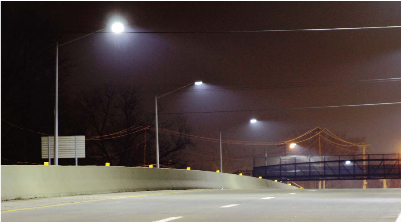
Dialight's StreetSense™ LED Street Light's reflector based optics direct the light to where it needs to be on the street
