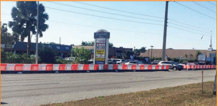
Longitudinal Channelizing Device Use on Roadways Instead of Traffic Barrels
