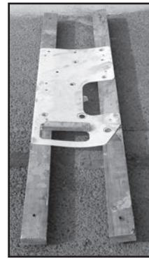
Example Concrete Template Chassis base & conduit
