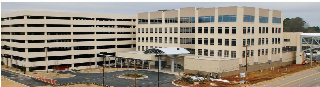
The eight-floor, 676-space garage was phase one of a five-phase hospital expansion. Photo courtesy of ComNet
