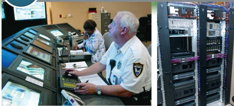
Left: The advanced security command center at the Jackson-Madison County Hospital. Right: Server equipment rack for the installation.
